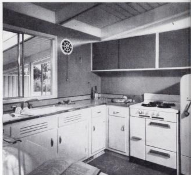
Not so long ago kitchen equipment like refrigerator, range, garbage grinder, and exhaust fan would have been considered extra furnishings to be provided by the buyer. But the price of this house covers all of them as well as well-planned kitchen storage and Formica counter tops.
