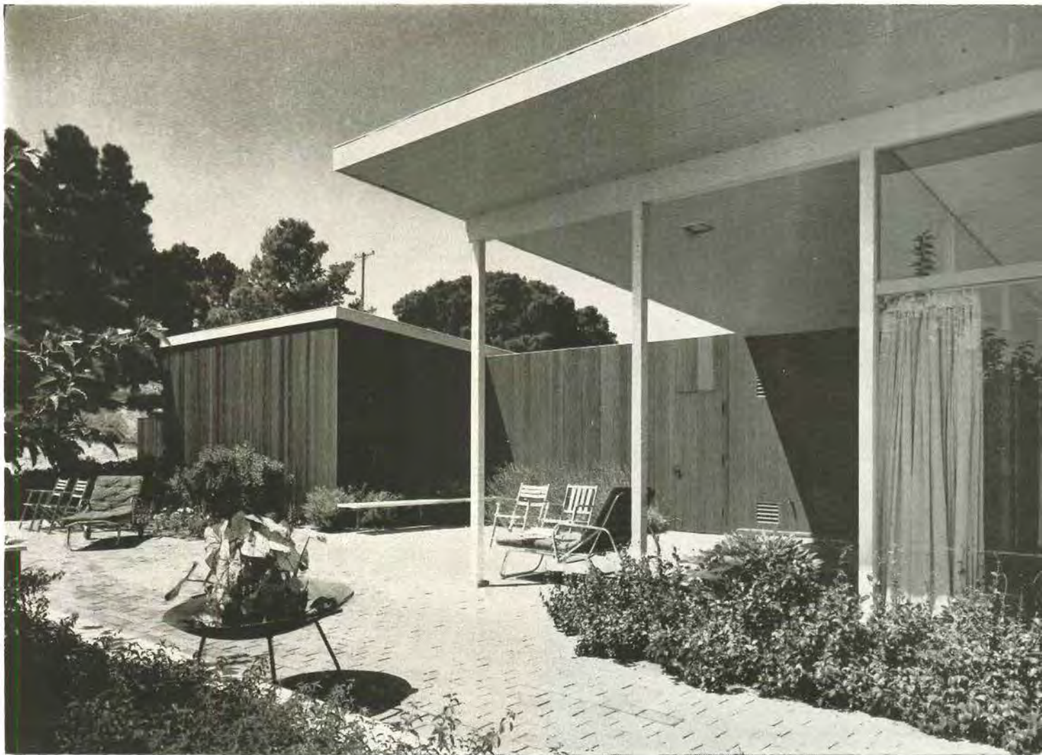
Picture below shows sunny court between garage wing and daytime living areas (see plan). Redwood screen wall to the north shields it from the service court. Dining porch is easily accessible from the kitchen. Paved area wraps around south facade of living wing, forms 100' long sun terrace. Glass walls along living area are 10' high.
