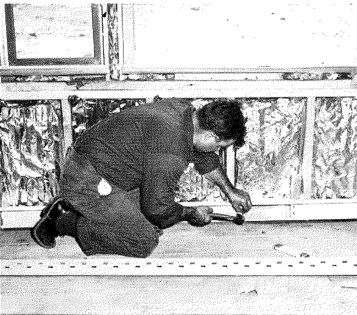
Metal baseboards can be used with wet- or dry-wall construction, are installed under all or most of outside walls depending on heat needs.
