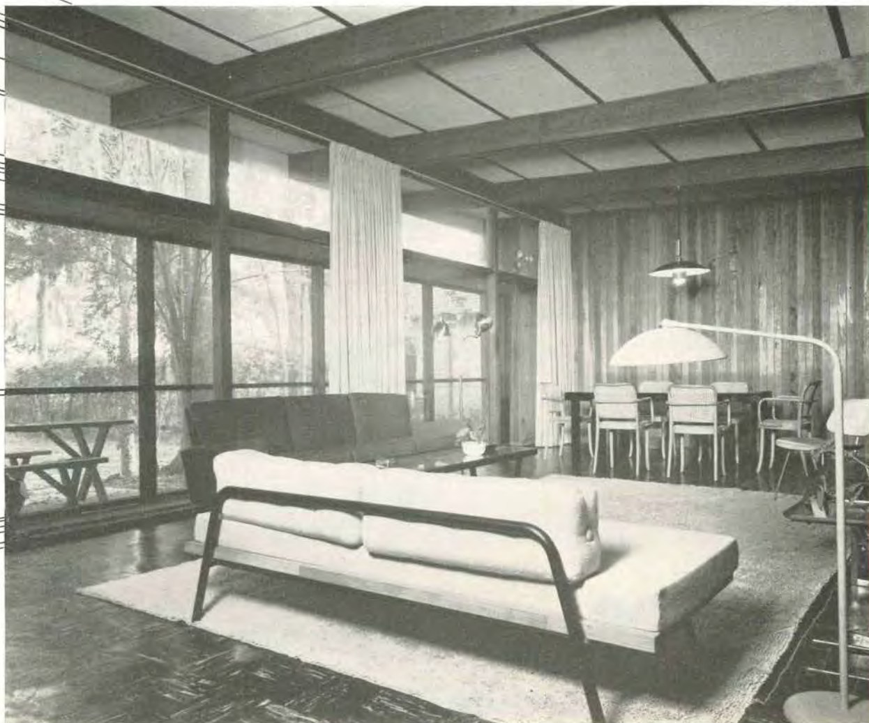
The roof structure is clearly visible in this picture: double redwood beams, steel purlins, cement and wood fiber board which also serves as the roof deck. Space between the screen cage and the sliding sash is part terrace, part plant bed.
