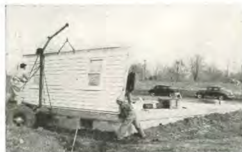
Builder who buys full-width panels with siding and windows may use mechanical cranes or large crews to install them.
