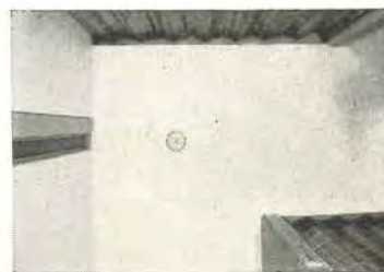
View of kitchen ceiling
