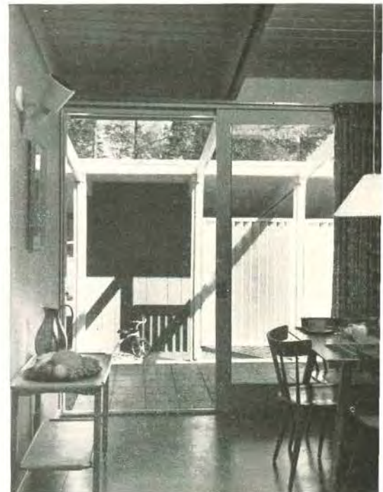
Opposite view from upper left photo. This shows how vertical louvers on the carport create a baffle from light, shutting out sight of automobile and creating a more filtered entrance. Open roof framing beyond door ties dining and garage together yet lets in light.
