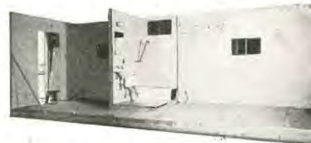
General Industries has gone further than most in building plumbing and fixtures into its low-cost demountable house.
