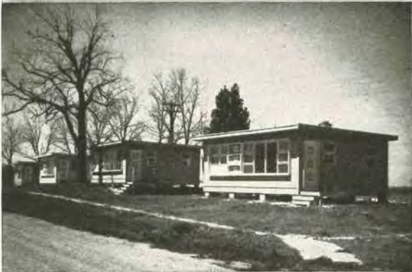
General Industries built 86 demountable 500 sq. ft. houses near the Kingsbury Ordnance Plant in Indiana.
