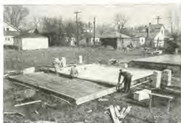
National Homes sells its dealers an easily installed, one-piece moisture barrier to cover the slab.
