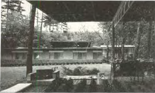
Bedroom wing seen from picnic pavilion
