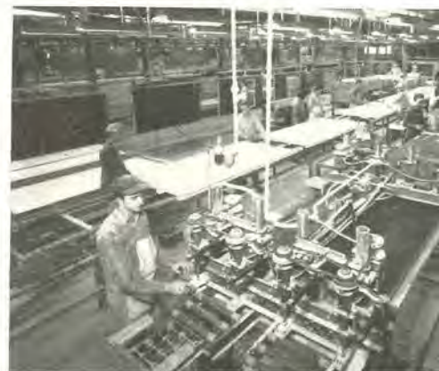
Automatic machines drill all bolt holes required wall panel in one operation. Production line, seen the background speeds completion of panels.
