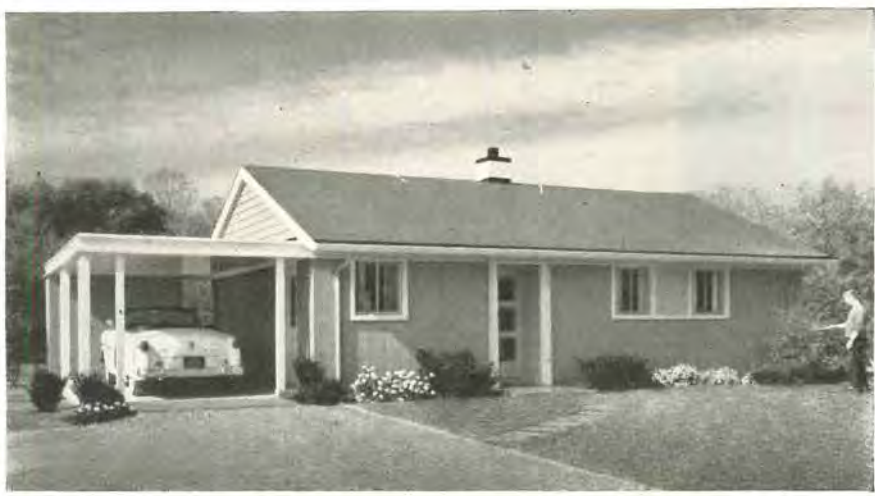
"195X" research house at Mequon, Wis. (plan, right & photo, p. 93 by architect John Normile. It has open plan, rear living areas and rear bedroom to go on narrow lots.
