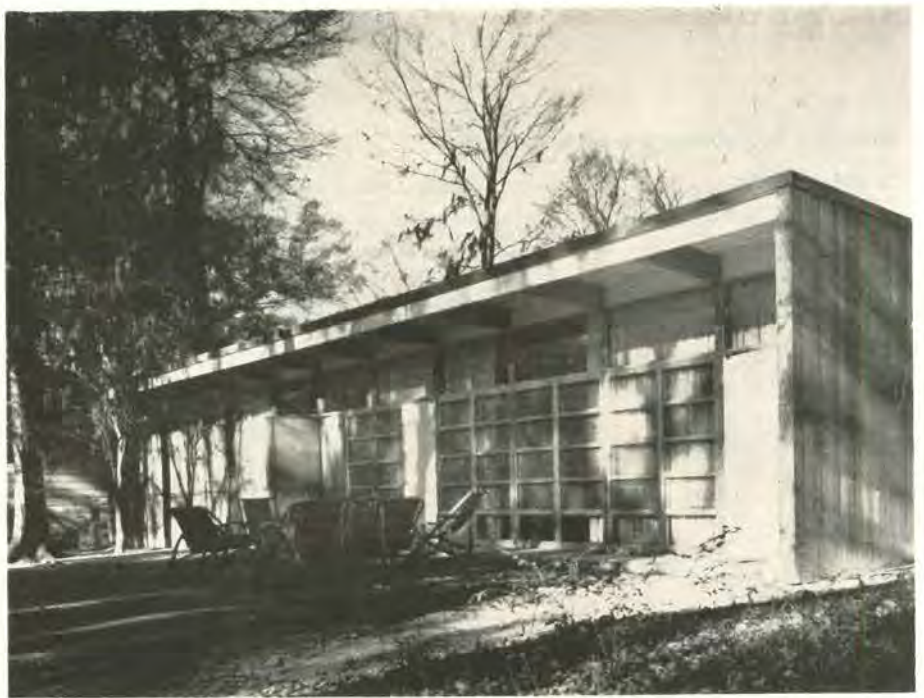
Oriented to the prevailing breeze, the rear of the house faces southeast toward the broad, wooded end of the triangular lot. This entire facade is glass, with awning-projected windows for the bedrooms, sliding sash for the living-dining area.
