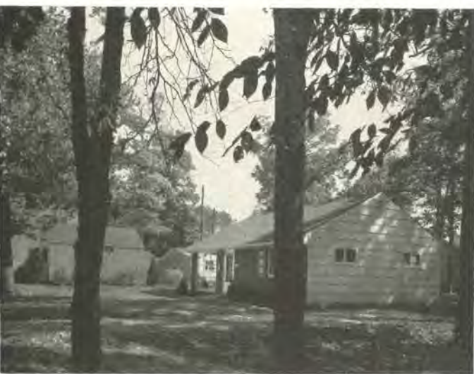
Co-ceiling window, brick front, wide overhang mark General Industries house, which is set well back from street, framed by tall trees.
