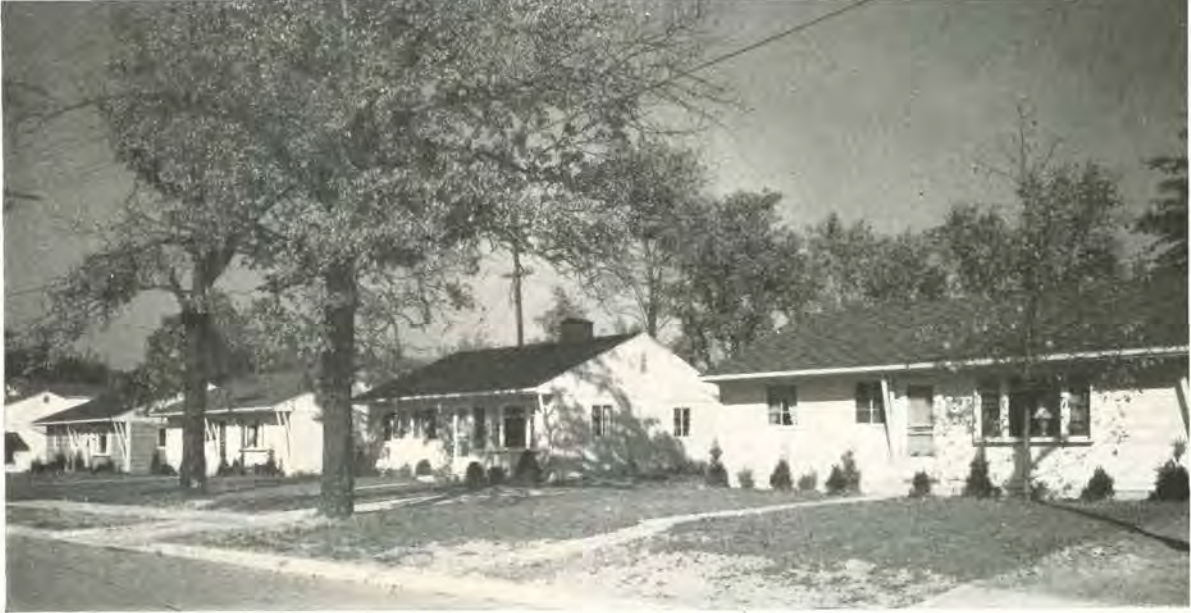
Row of Gunnison houses gains some variety in different colored roofs, changes in type and of siding. Looking at these houses Gunnison dealer Hamilton Hunter says that prefabrication need not be disguised.
