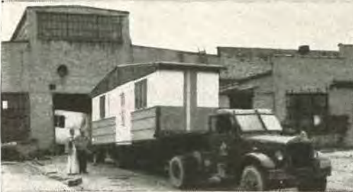
This Knox-Bergstrom fold-out telescopes into a complete package. A transportable three-dimensional unit is formed by two adjacent units. . . .
