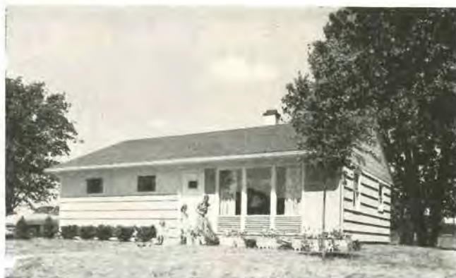
Current "Saratoga" has vent louvers, double glazing
