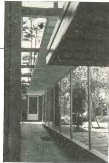
Approach between garage and service wing
